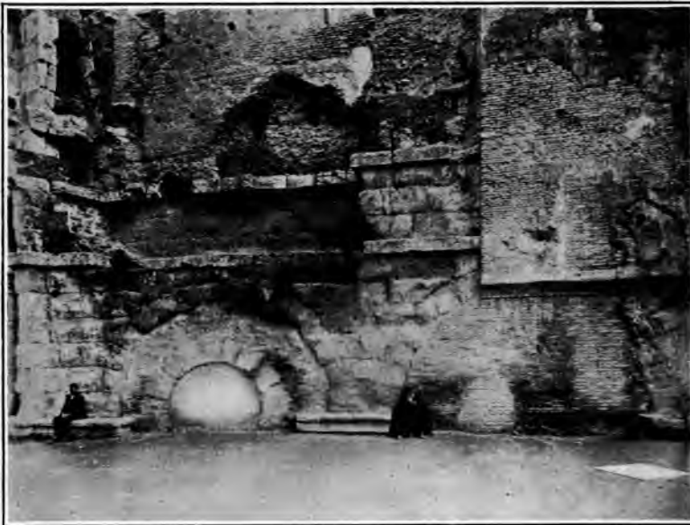
FIG. 2. — Marcia, Tepula, and Julia Aqueducts, near Rome.
